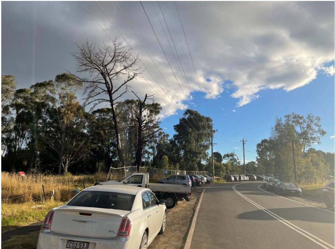
Phot. 4. Endeavour Energy HV power lines on Croatia Av. north-east of the property.
