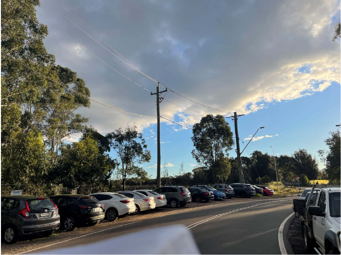
Phot. 3. Endeavour Energy HV power lines on Croatia Av. at the intersection with Soldiers Pde.
